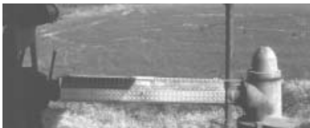
Figure 12-2. Install shields to protect anyone working around well power shafts.
