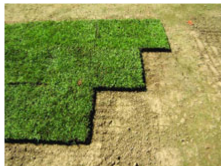
Figure 4. On each row of sod, stagger the joints as when laying bricks.
