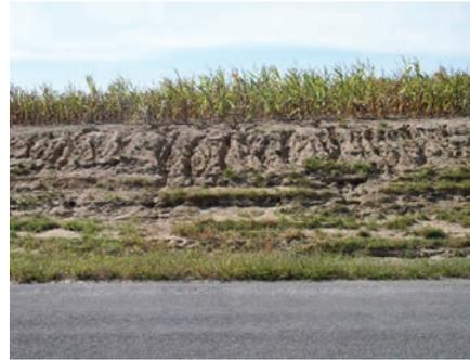
**Figure 2. Soil erosion along a ditchbank lacking grass groundcover.**
