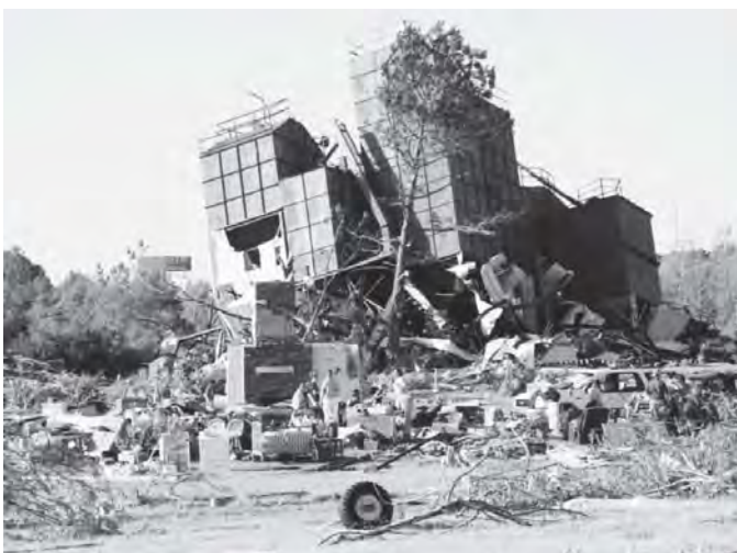
Figure 2. Tornado damage in Damascus, Arkansas, on May 2, 2008.
