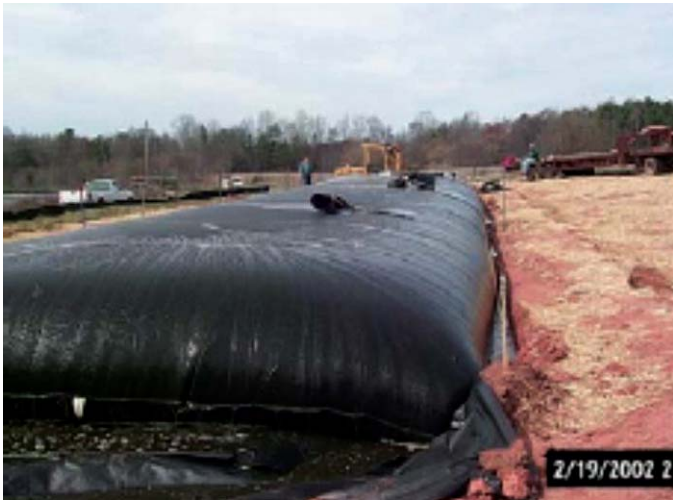
Figure 2. Fabric dewatering tube after it has been loaded.
