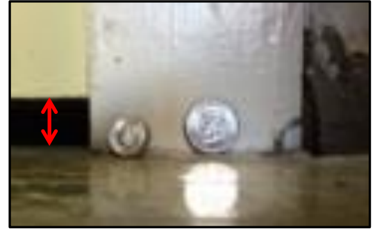
A mouse or rat could easily slip under this door
