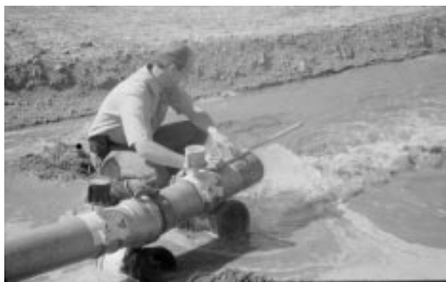
Flow meter and plumb bob measurement of water flow in a horizontal pipe from a riser.
