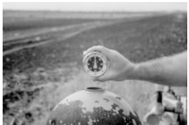
A portable tachometer being used to check turning speed of gear-head and pump.
